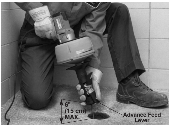
Figure 10 – Feeding Cable With AUTOFEED
