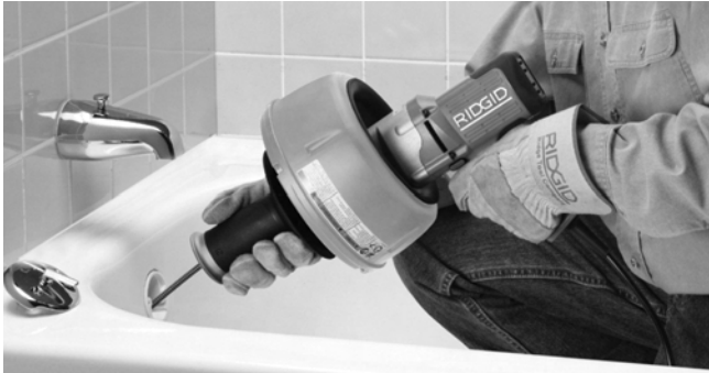
Figure 9 – Push Cable Down Drain Line
